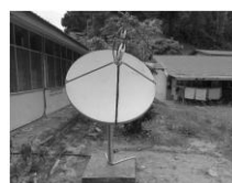
VSAT dish ground installations
