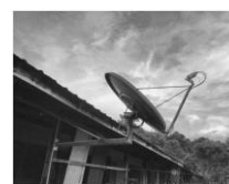
VSAT dish wall-mounted installations
